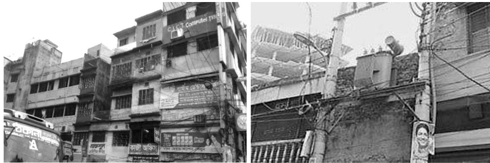
Fig. 4. Image of buildings without any space between each other (left image) and placement of transformer near residential building (right image) in Nimtoli area.
